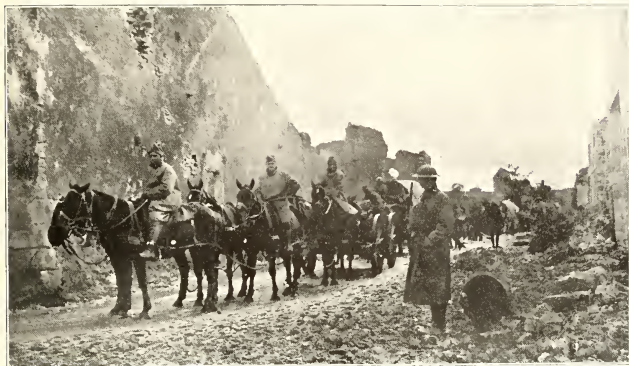
SUPPLY TRAIN OF THE FIRST ENGINEERS, MOVING THROUGH THE DEVASTATED AREA NEAR THE OLD FRONT LINE NORTH OF VERDUN
